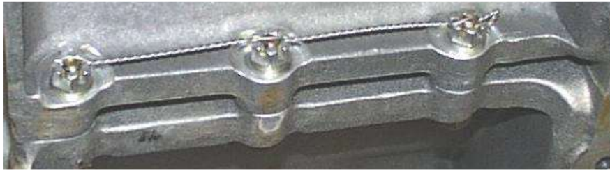
Figure 91 Safety Wire Nuts in Crankcase Oil Sump
